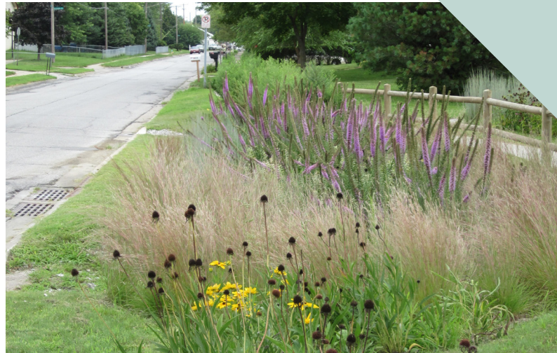
Rain gardens and bioswales, like this one in Omaha, capture and clean water before it enters a stream.
