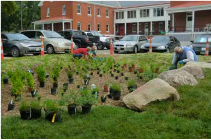
Bioretention garden at Metro Community College in Omaha
