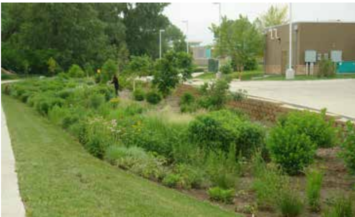
Bioswale at Fireworks Restaurant in Lincoln
