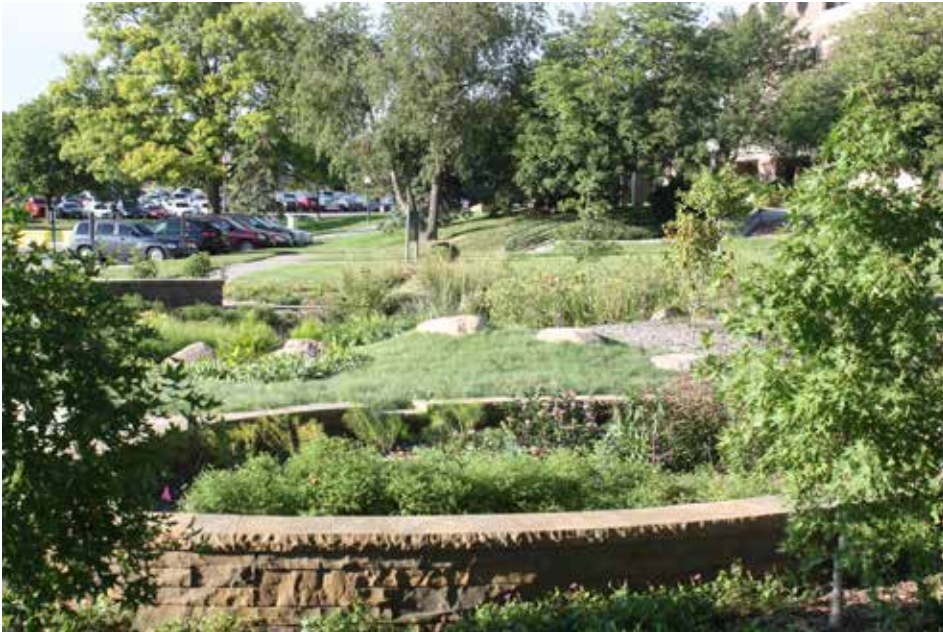
Omaha is working hard to slow down and capture rainwater. Above: UNO Welcome Center Bioretention Garden.
