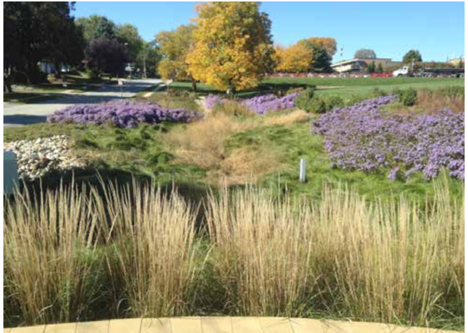
Above: Saddle Hills Rain Garden.
