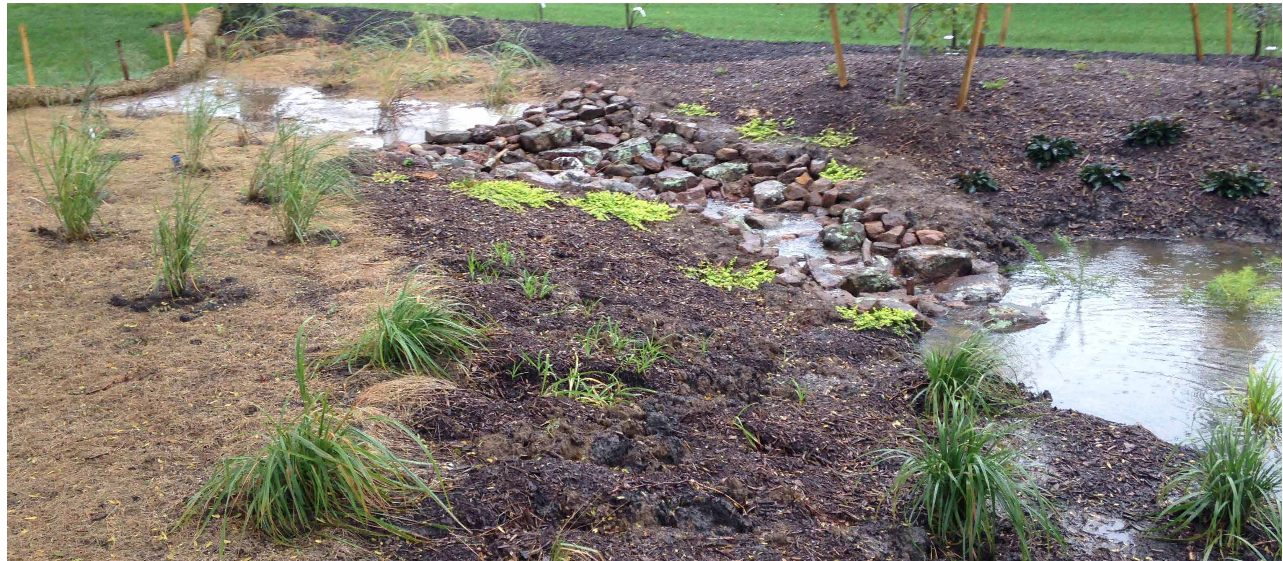
The raingarden functioning during a rain event. It took a few rounds of modifications to get it to drain right.
